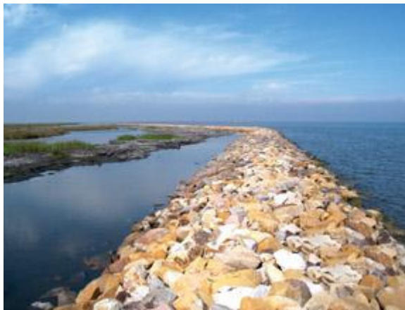
ROCKS SOLID: A rock dike barrier, built at Little Lake in Lafourche Parish, works to protect coastal wetlands and slow erosion.
